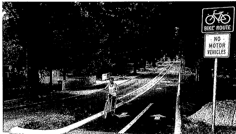
Figure 5: Tremain Street Greenway in Mount Dora
